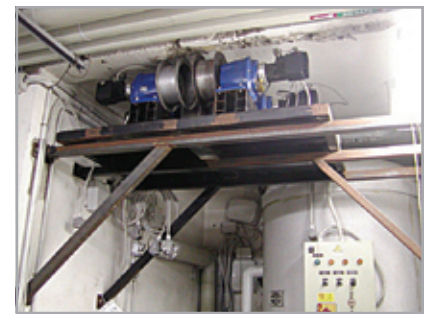
Two of the installed MAC800 motors
